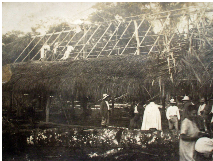
FIGURE 3 Constructing the School Building at Casarabe
