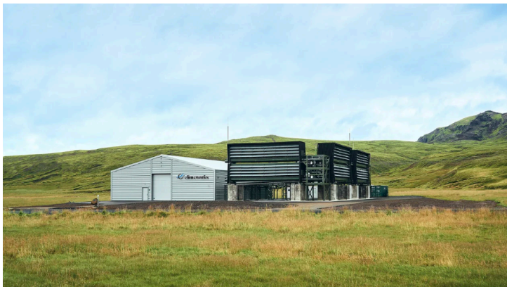
Figure 5. Climeworks building in the countryside.
