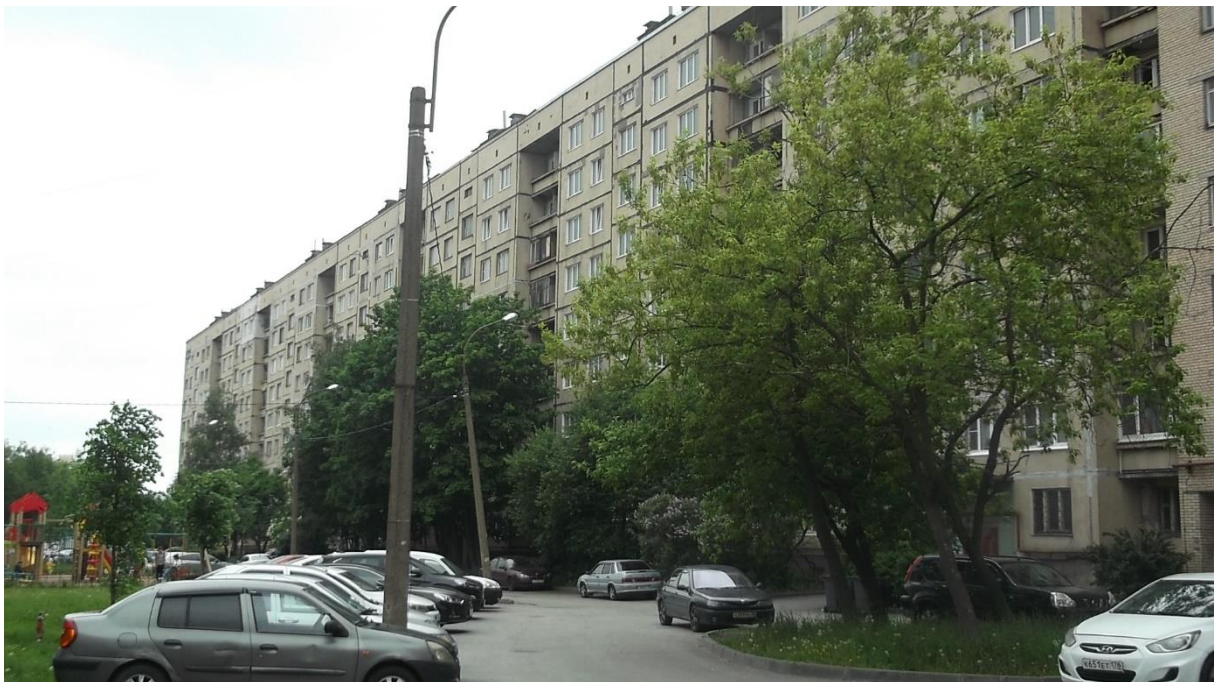
Figure 12. Nine-storey Brezhnevka in the district of Frunzensky, Saint Petersburg, May 2020. Following the aesthetical example of Khrushchyovkas, Brezhnevkas were minimalistic and based on the repetition of prefabricated modules. Own photo.
