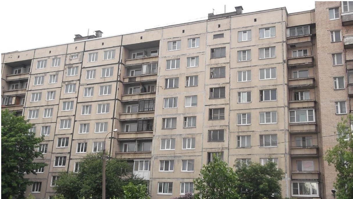
Figure 11. Nine-storey Brezhnevka in the district of Frunzensky, Saint Petersburg, May 2020. This kind of constructions was built in the mandate of Brezhnev, and thus, they were baptised after him. Own photo.
