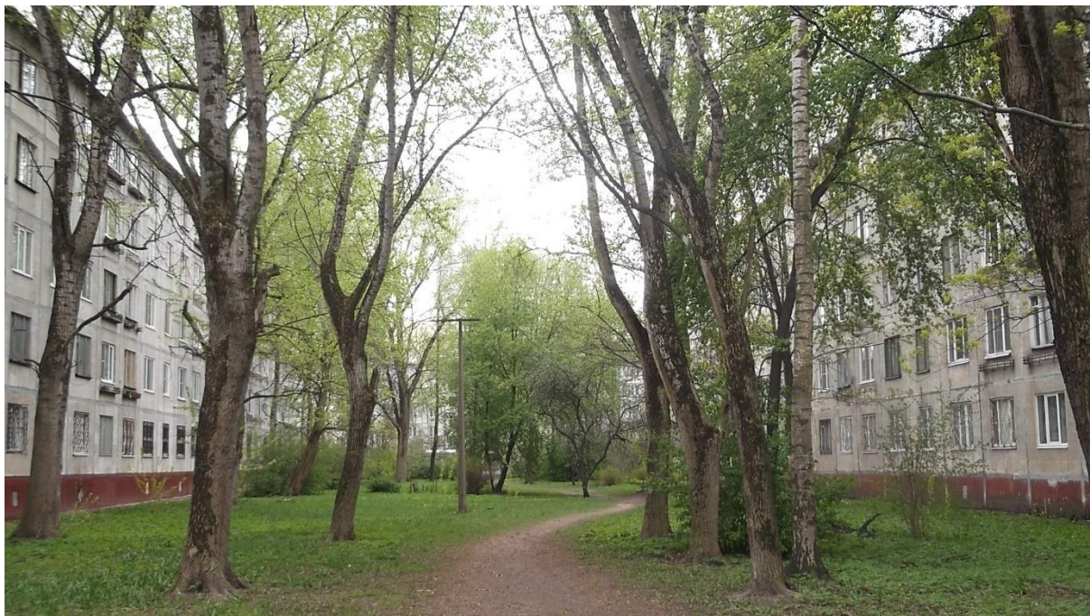
Figure 8. Five-storey Khrushchyovkas in the district of Frunzensky, Saint Petersburg, May 2020. A great part of this district is made up of these identical Khrushchyovkas, making the landscape monotonous. Own photo.
